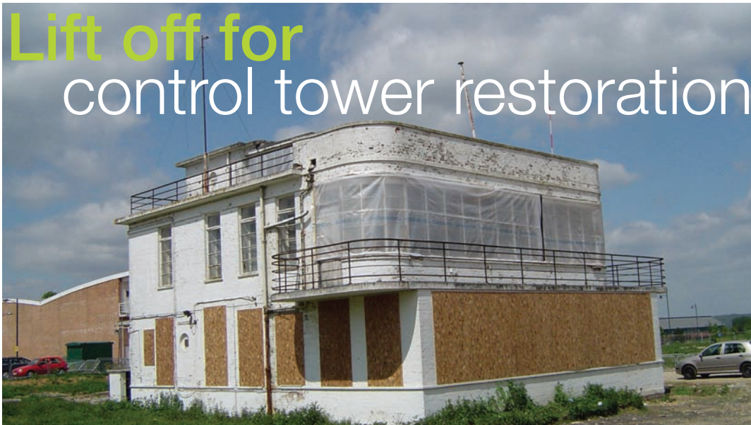
The control tower at West Malling Airfield
