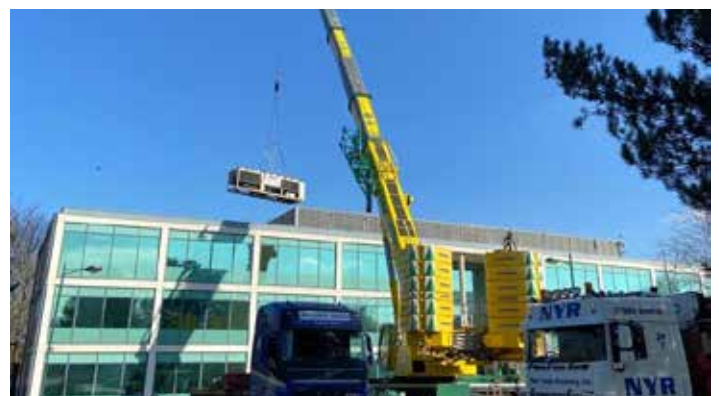
30 Tower View - new chiller crane lift
